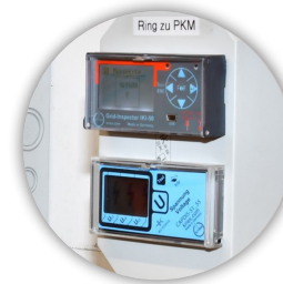
IKI-50 + CAPDIS (Directional Fault Detection)
